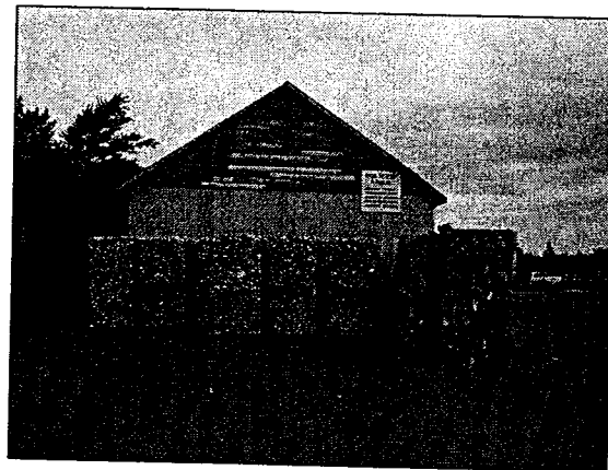
Photo No. 3 - South Side of Storage Building
