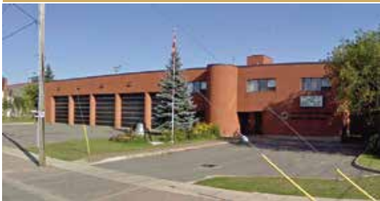
Station 1 - MAIN FIRE HALL
