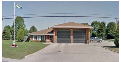
Station 3 100 Bennett Blvd.
