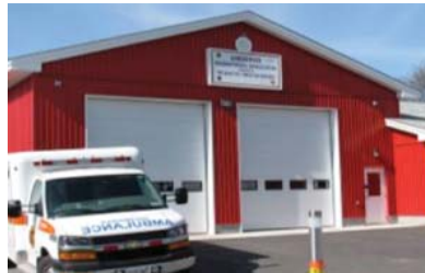
EMS-Garden River 15 Shingwauk Street
