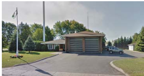
Station 2 363 Second Line West
