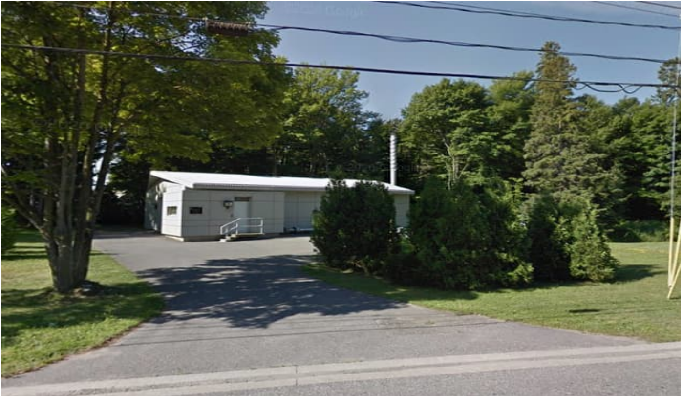
Clark Creek Lift Station
