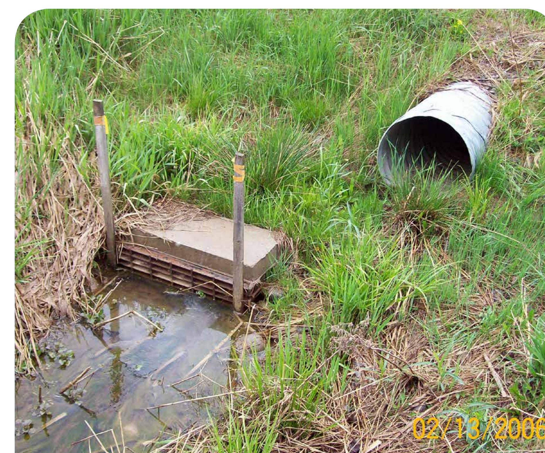
Stormwater Management Ponds - 11
