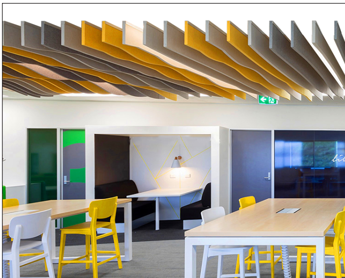
Ceiling baffles and acoustical tiles reduce the level of airborne sound.
